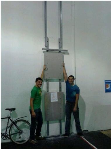
**Image 1:** The rectangular frame with mounting plates, bolted into the metal stud-wall in Apex Movement gym.
